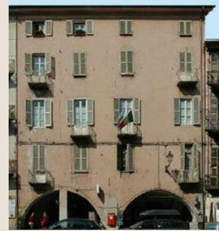
THE FAÇADE PRIOR TO THE RESTORATION
