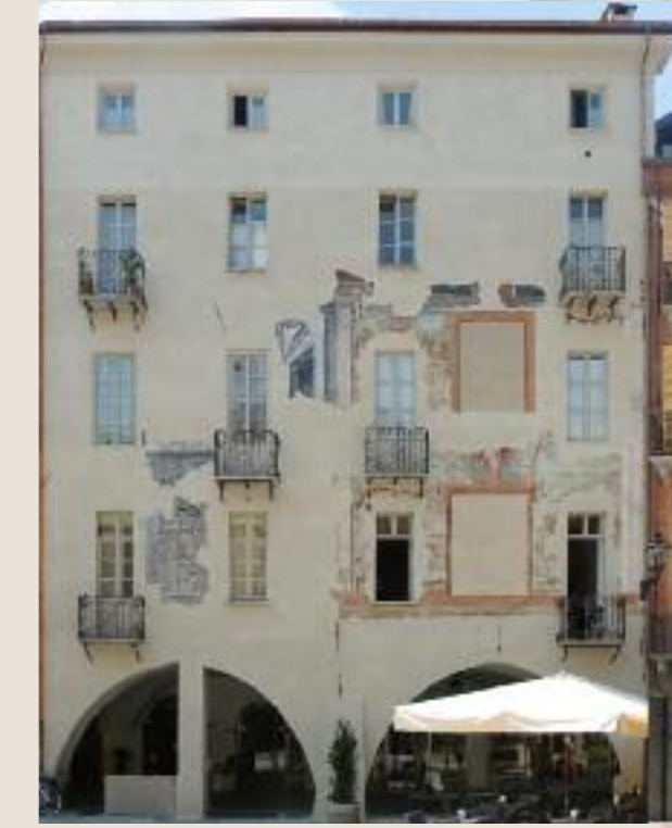
THE FAÇADE AFTER THE RESTORATION
